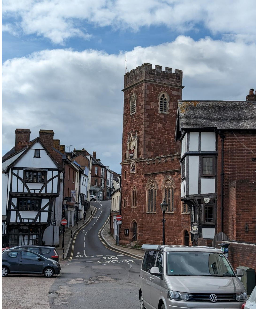
PHOTO OF EXISTING SITE FROM WEST 1
