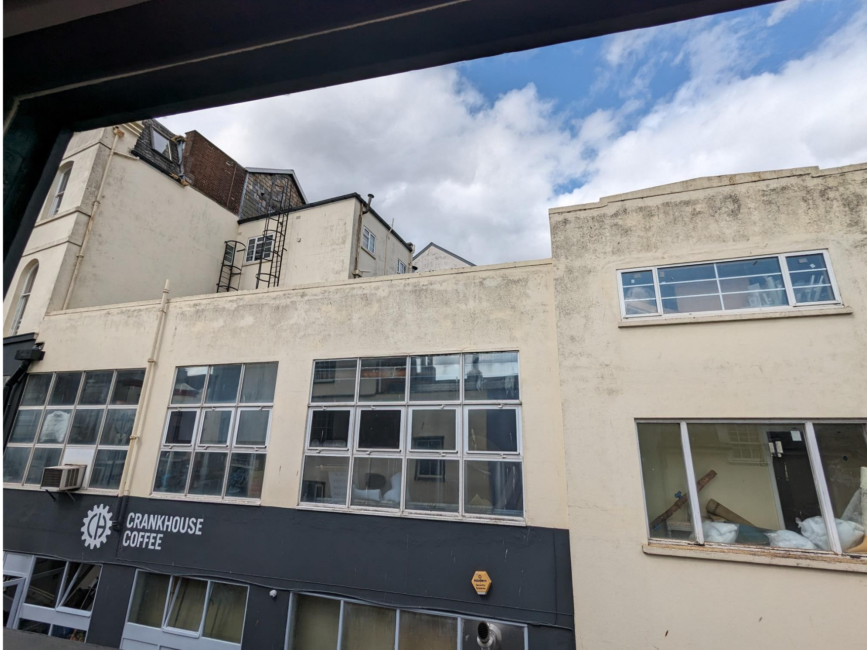
EXISTING VIEW FROM OPPOSITE WINDOW
