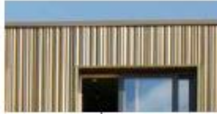
Bronze effect profiled metal cladding to link block & inset top floors.
