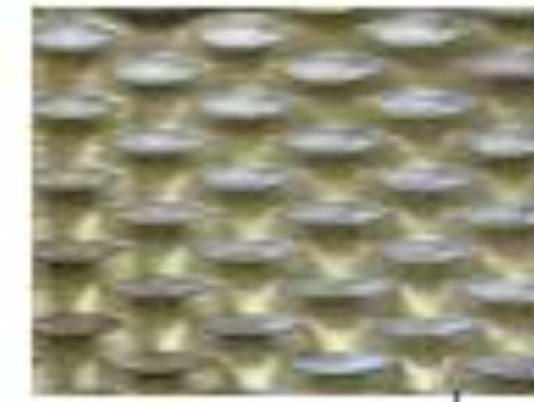
Perforated bronze effect screen to ASHP enclosure, set behind the brick parapet upstand.
