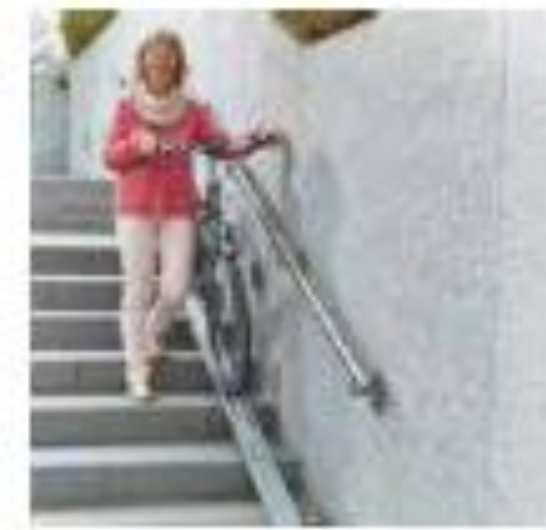
13D No Long stay cycle spaces within store at lower grd accessed via steps with integrated bike ramp
