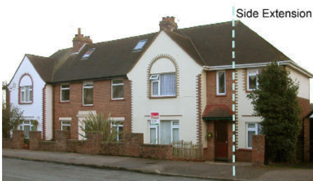
Figure 1.2 The above side extension is successful although it is not set below the original ridge or set back from the front elevation.
