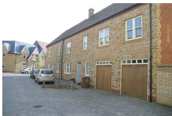
Figure 6.15 Well-designed garage doors integrated into the design of the buildings.
