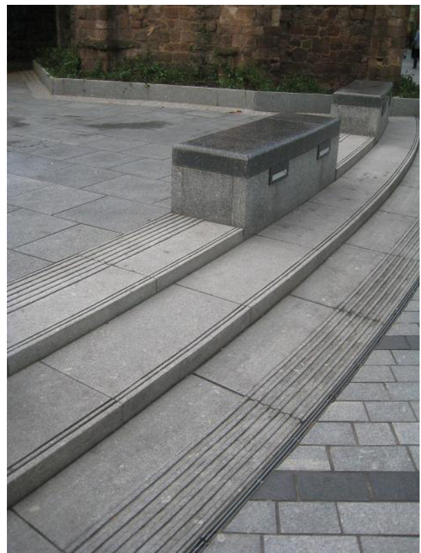
Figure 10.8 Carefully detailed granite steps and tactile paving.
