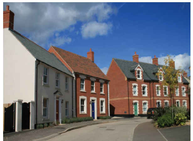
Figure 5.19 Attractive elevations uncluttered by meter boxes or satellite dishes.
