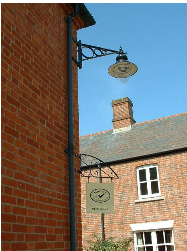
Figure 10.17 A Wall mounted street light.
