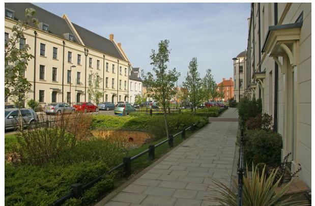
Figure 10.3 High quality paving and planting creates an attractive streetscene.
