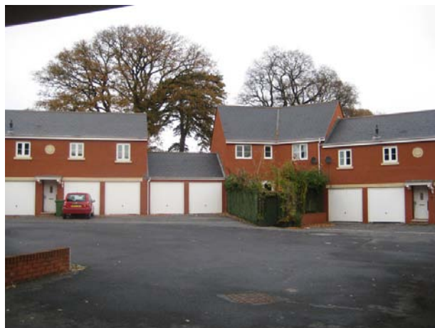
Figure 6.20 Lack of care with architectural and landscape design made this mews court an unattractive place.
