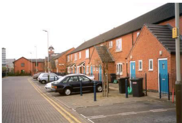
Figure 6.13 Right angled parking enclosed by two storey houses produces poor townscape.
