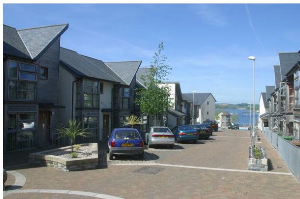
Figure 6.9 A recently completed homezone development.
