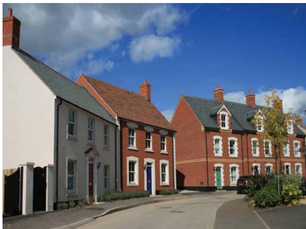
Figure 9.19 Traditional style buildings forming an attractive street scene.
