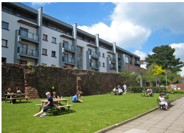
Figure 6.23 Good quality open space provided above underground parking.
