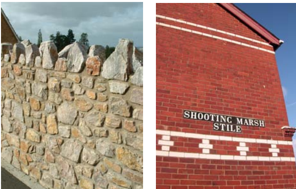
Figure 10.2 Local detailing helps to create a strong sense of place, such as this 'Cock and Hen' coping detail and Minton tile street-names
