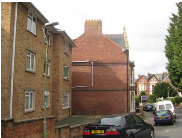
Figure 4.5 Jagged building lines result in unsatisfactory street scene
