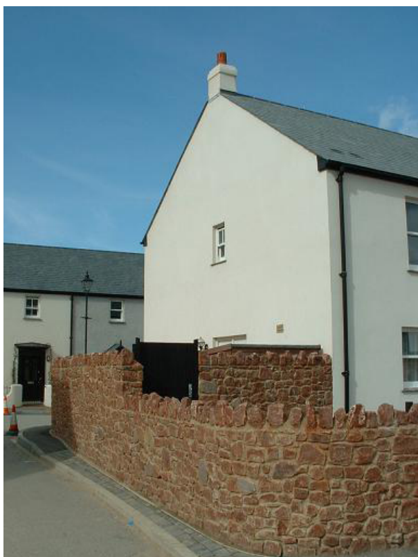
Figure 10.13 High quality local stone garden wall.
