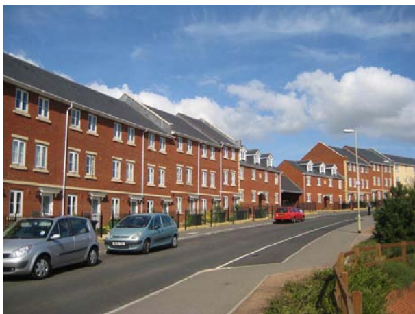
Figure 5.13 In this example the introduction of a change of house type has spoiled the crescent effect and demonstrates the importance of consistent building form.
