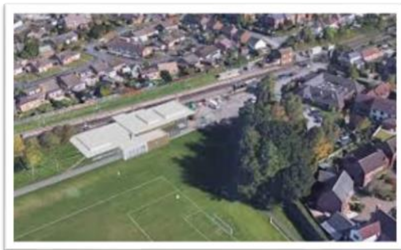
Image 7: the location of the proposed Pinhoe Community Hub on the Station Road Playing Fields
