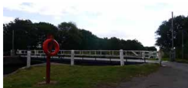
Salmonpool swing bridge
