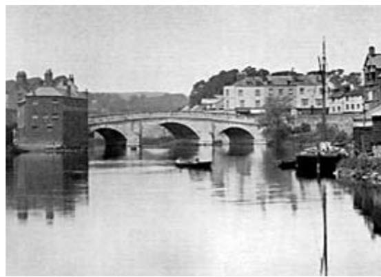
Georgian Exe Bridge
