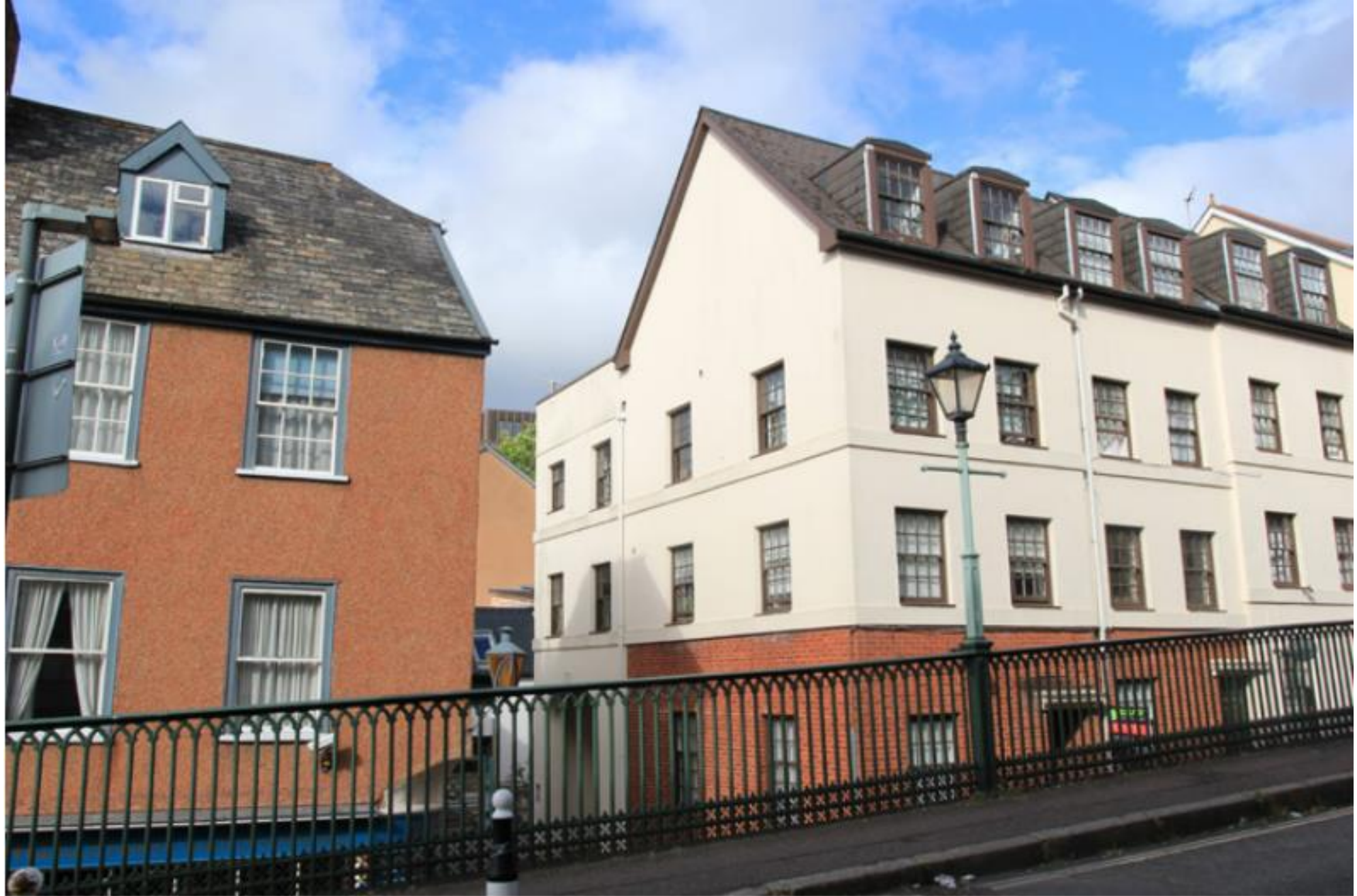
LVA VIEWS – IRON BRIDGE
