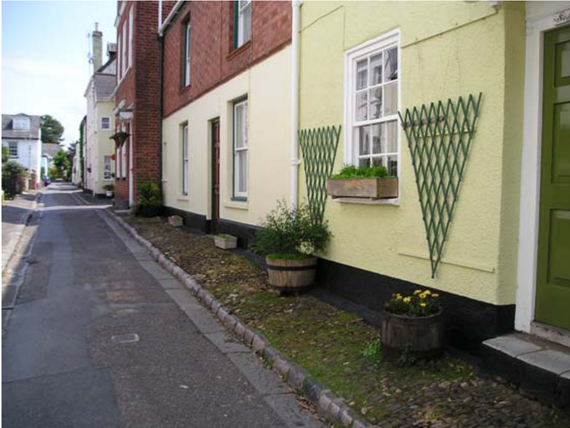
Higher Shapter Street, displaying the cobbled pavement, limestone kerbs and gullies
