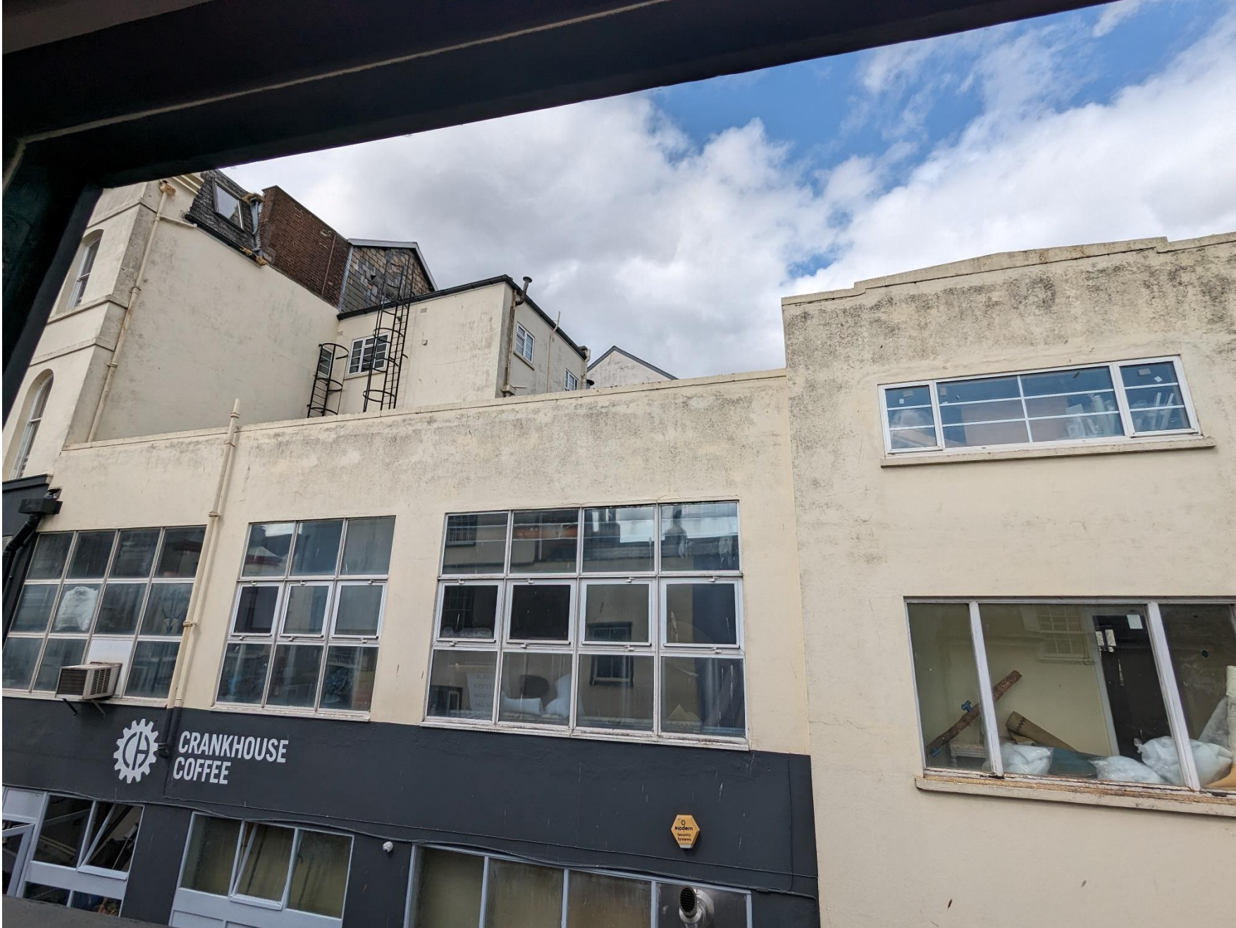
EXISTING VIEW FROM OPPOSITE WINDOW
