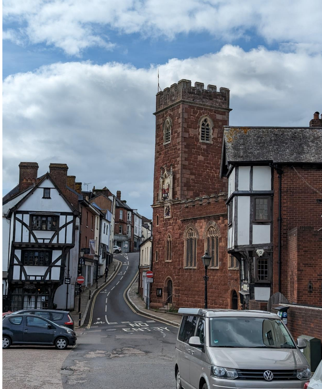
PHOTO OF EXISTING SITE FROM WEST 1
