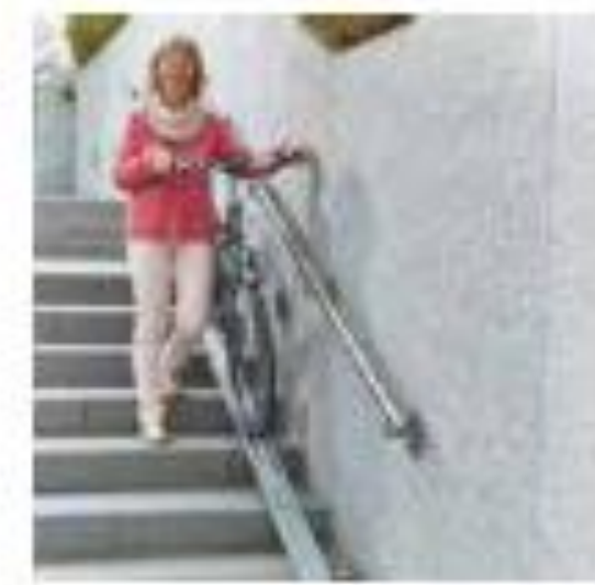
13D No Long stay cycle spaces within store at lower grd accessed via steps with integrated bike ramp
